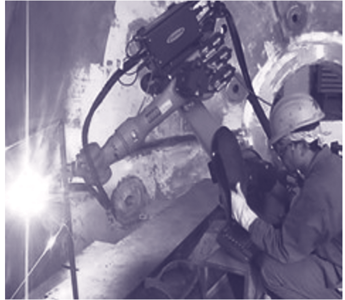
Figure 5: Robotic Clad Restoration in Action
